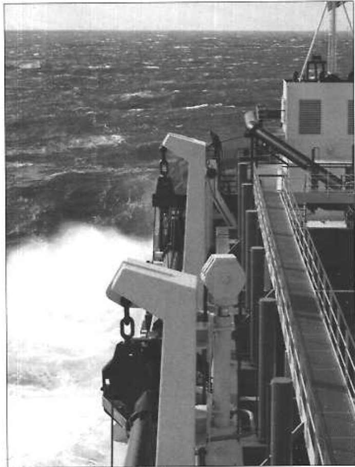
View on the lowered port suction pipe
