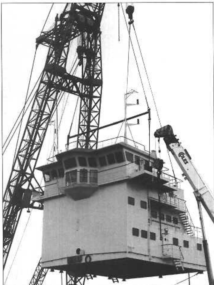
The pre-fabricated deckhouse section is lifted into its position.
